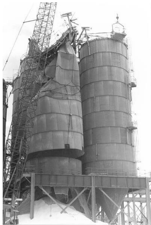
Fig. 5, End-result of mass flow developing in a silo designed structurally for funnel flow
