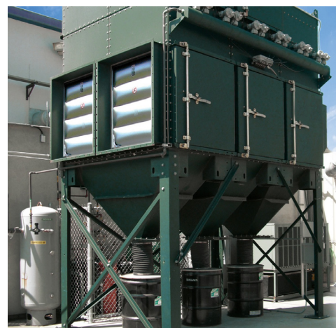
Industrial dust collector with explosion venting
