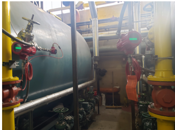
Figure 2. Flowmeters help engineers “tune” boilers to maintain the optimal efficiency, which minimizes greenhouse gas emissions
